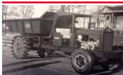
1934 The model 1Z truck- considered to be the first true off-highway rear dump truck.
