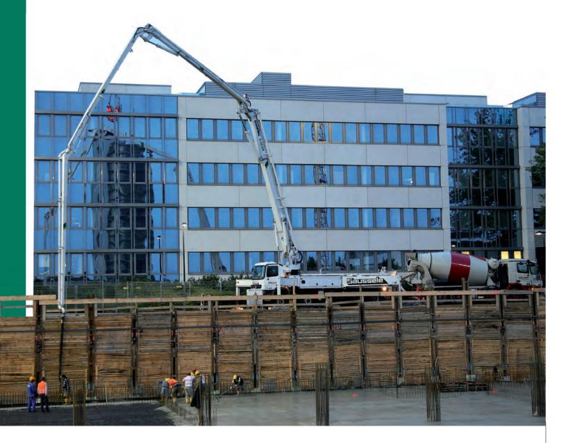
Plus, the SCHWING long-stroke pump kit cuts energy consumption and friction resistance further by using smaller reductions between the material cylinder and the valve system. This makes for significantly less wear. Together with the Rock Valve system and the open hydraulic circuit, this means higher energy efficiency and greater economy of SCHWING concrete pumps.
