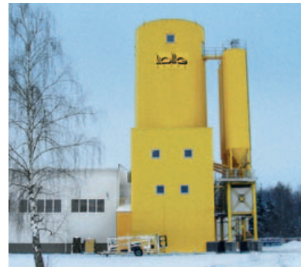
Thermal insulation of mixing and weighing platform is done with sandwich or profiled plates/mineral wool/smooth plates. The section \pm 0 up to the lower edge of the platform can optionally be covered. For thermal insulation of the aggregate silo profiled plates/mineral wool will be used.
