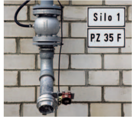
The safety device to prevent overfilling of the cement silo meets the requirements of the UVV. A squeeze valve in conjunction with an optional pressure controller prevents overblowing of the cement silo.
